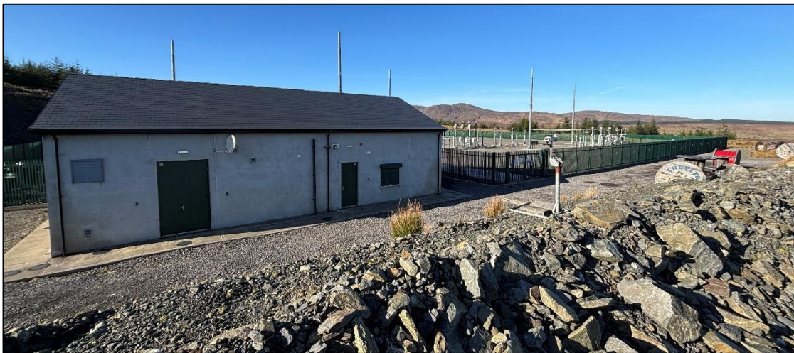
Plate 13-7 View facing northwest towards the Substation
